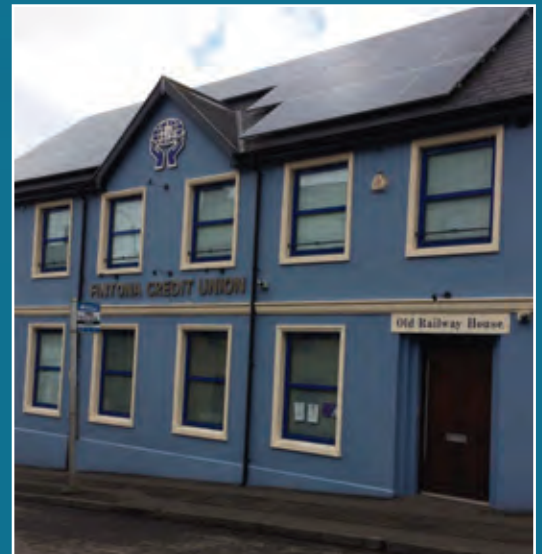
Fintona Credit Union Offices
