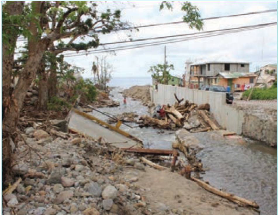
Infrastructure damage following Hurricane Maria
